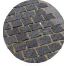
P2: UNIT PAVEMENT TYPE 2 Granite paving bands within concrete paving to define Waterfront Plaza
