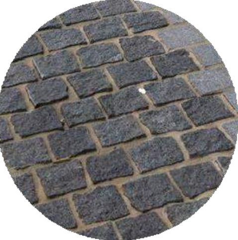
P2: UNIT PAVEMENT TYPE 2 Granite paving bands within concrete paving to define the shared zone in Market Square
