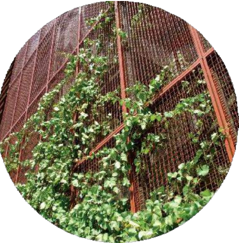
ENTRY WALLING Steel frame growing trellis to screen carpark.
