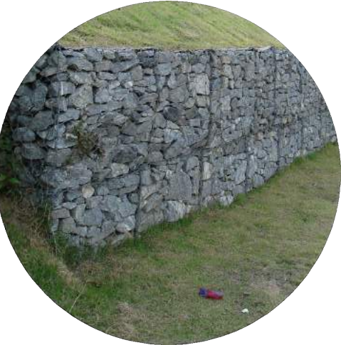
ENTRY WALLING Gabion wall to screen car park.
