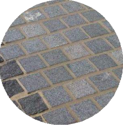
P1: UNIT PAVEMENT TYPE 1 Granite paving bands within concrete paving.
